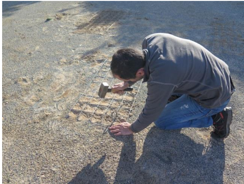
Photo 7. Example of a metal grid fixed to the ground
